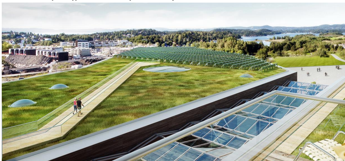
The combination of heat from the fjord, environmentally friendly materials, low-CO2 concrete, plenty of insulation, green roofs, the solarcell panel park on the roof and good environmental-planning processes has led to the Area Centre at Fornebu being certified as Outstanding by BREEAM. Photomontage: KLP Eiendom.
